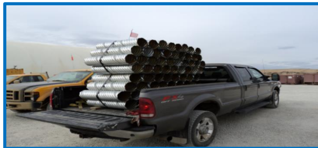
Materials are not supported on pallets for easy off-load.
