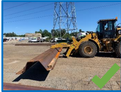
Grapple attachment handling sheet piles.
