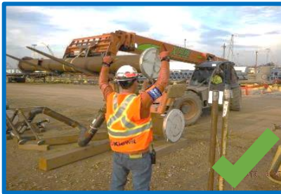
Grapple attachment handling sheet piles.
