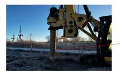
Kelly Bar, when pulled all the way up, sections are all fully retracted. In this photo the inner bar is retracted below the outer section.
